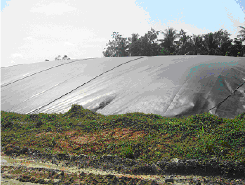
The anaerobic digester with HDPE cover. Biogas is already trapped inside.
