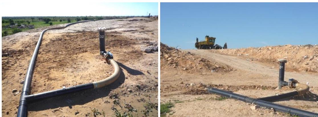
Figure 8. Piped vertical wells of the gas collecting network
