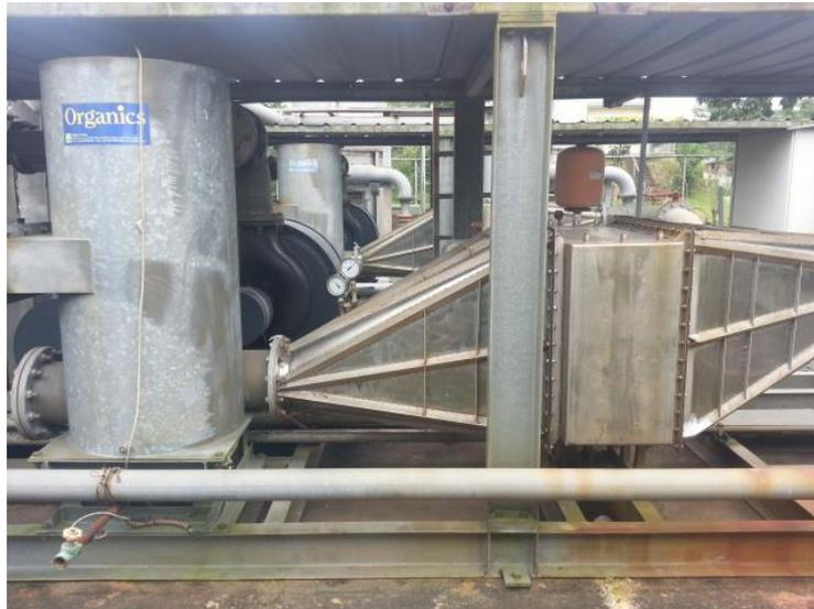
**Figure 11. Heat exchanger and condensate knock-out pot**
